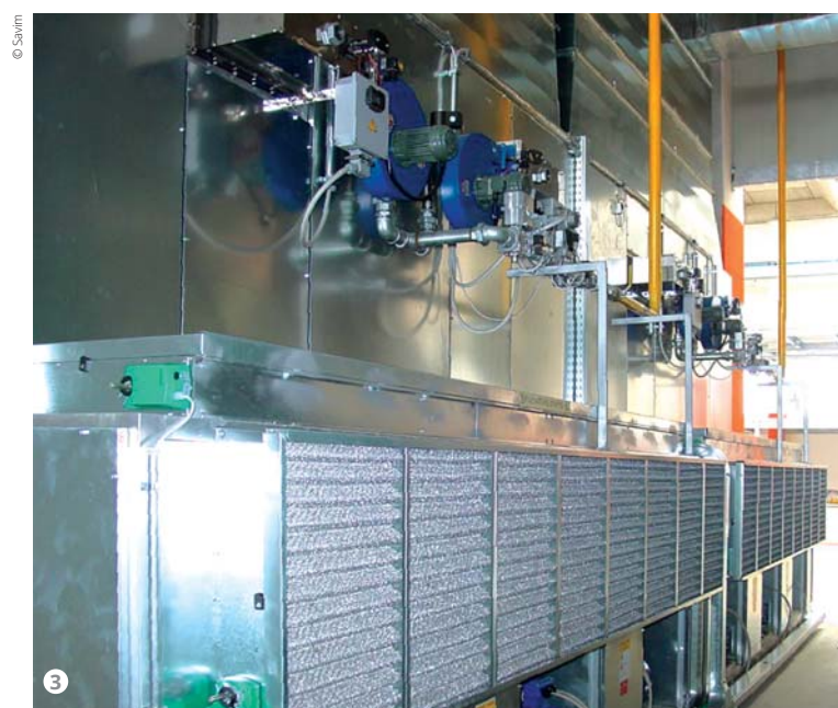
Figure 3: Direct fire heating units for Savim’s coating booths.
