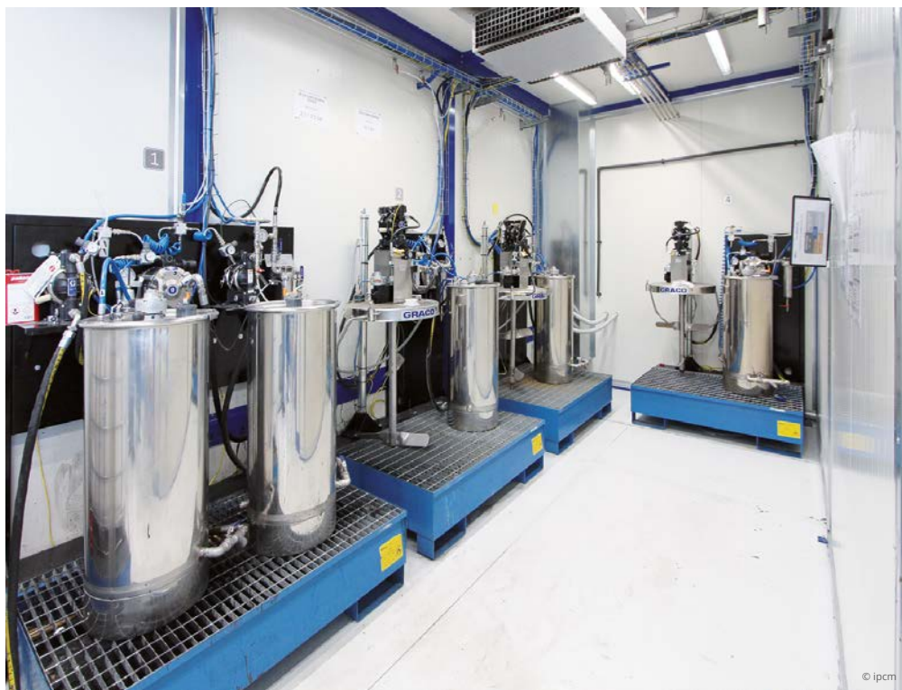
The paint management unit set up by Comaind with Graco Endura-Flo pumps.
