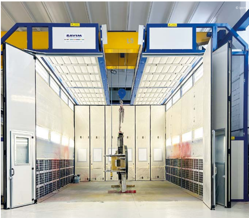
Savim Europe's coating booth, divided into three sections.
